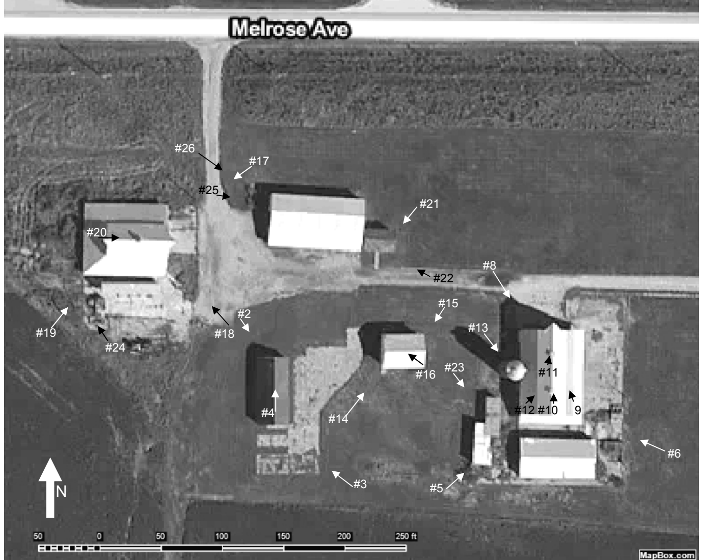
2013 Aerial map showing direction of photographs #2-6, #8-26 of Johnson County Poor Farm and Asylum buildings and structures. Source for base aerial: 2013 aerial photograph obtained from ExpertGPS mapping software, 2014
