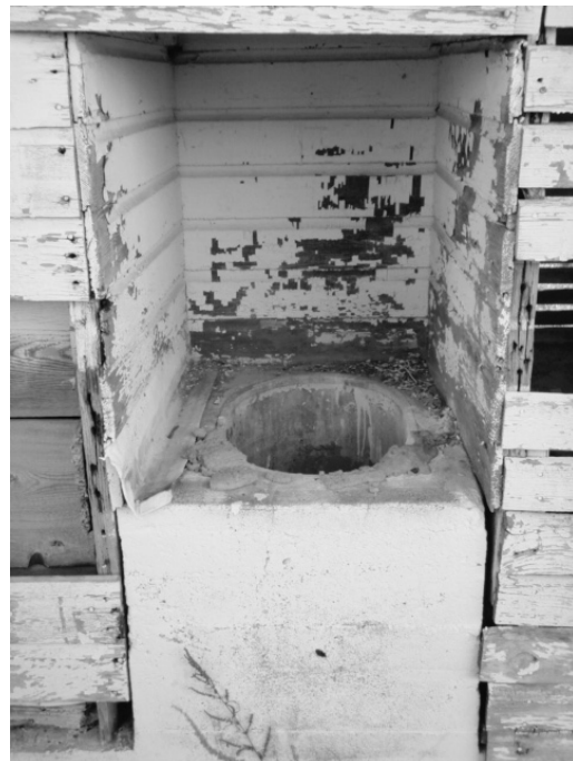
Metal basin built into east side of Crib
