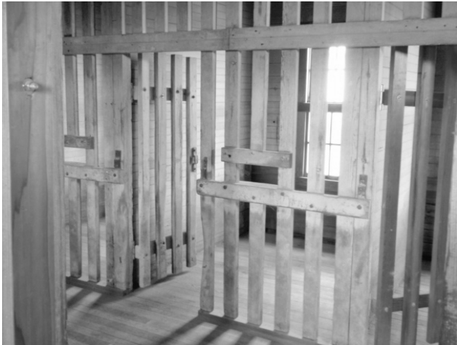
Cell in Asylum showing original and restored framing
