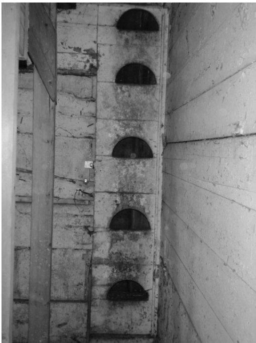
Original hand-held ladder built into south wall of Dairy Barn
